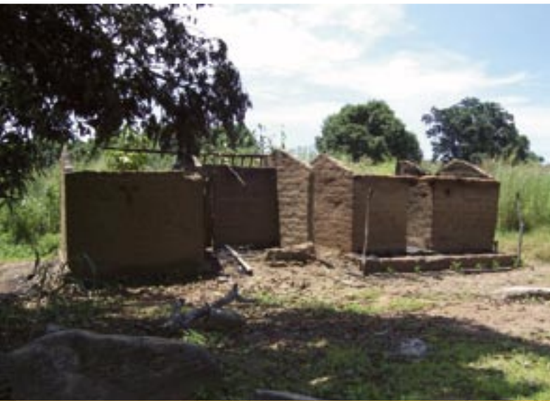
Destroyed houses in northern Central African Republic. (Photo: Mpako Fোলeng, IDMC)
