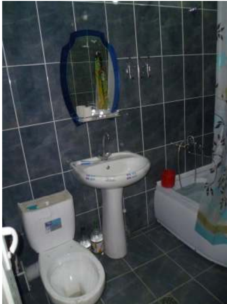
Rehabilitated bathroom property number 25
