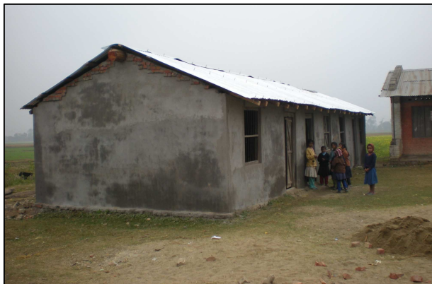
Figure 1 : Rastriya Primary School before and after support in Kailali- Photo SC
