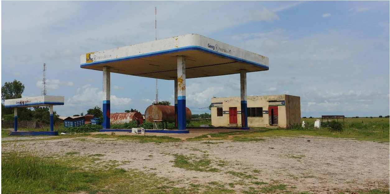
Figure 1 An abandoned petrol station in Bentiu Town
