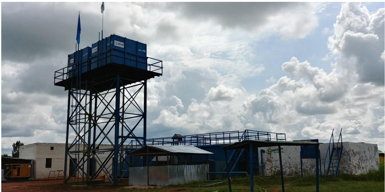
Figure 3 A water distribution center in the town provided by humanitarian organizations
