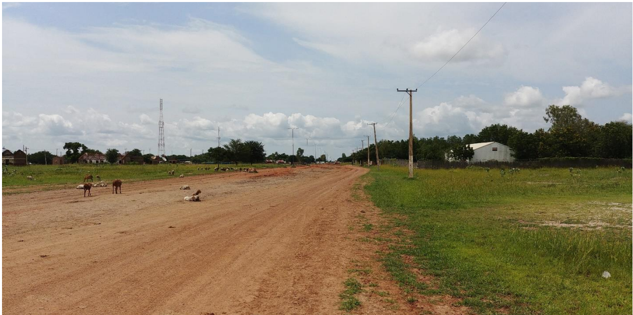
Figure 2 Electrical wires line the main road but no longer function
