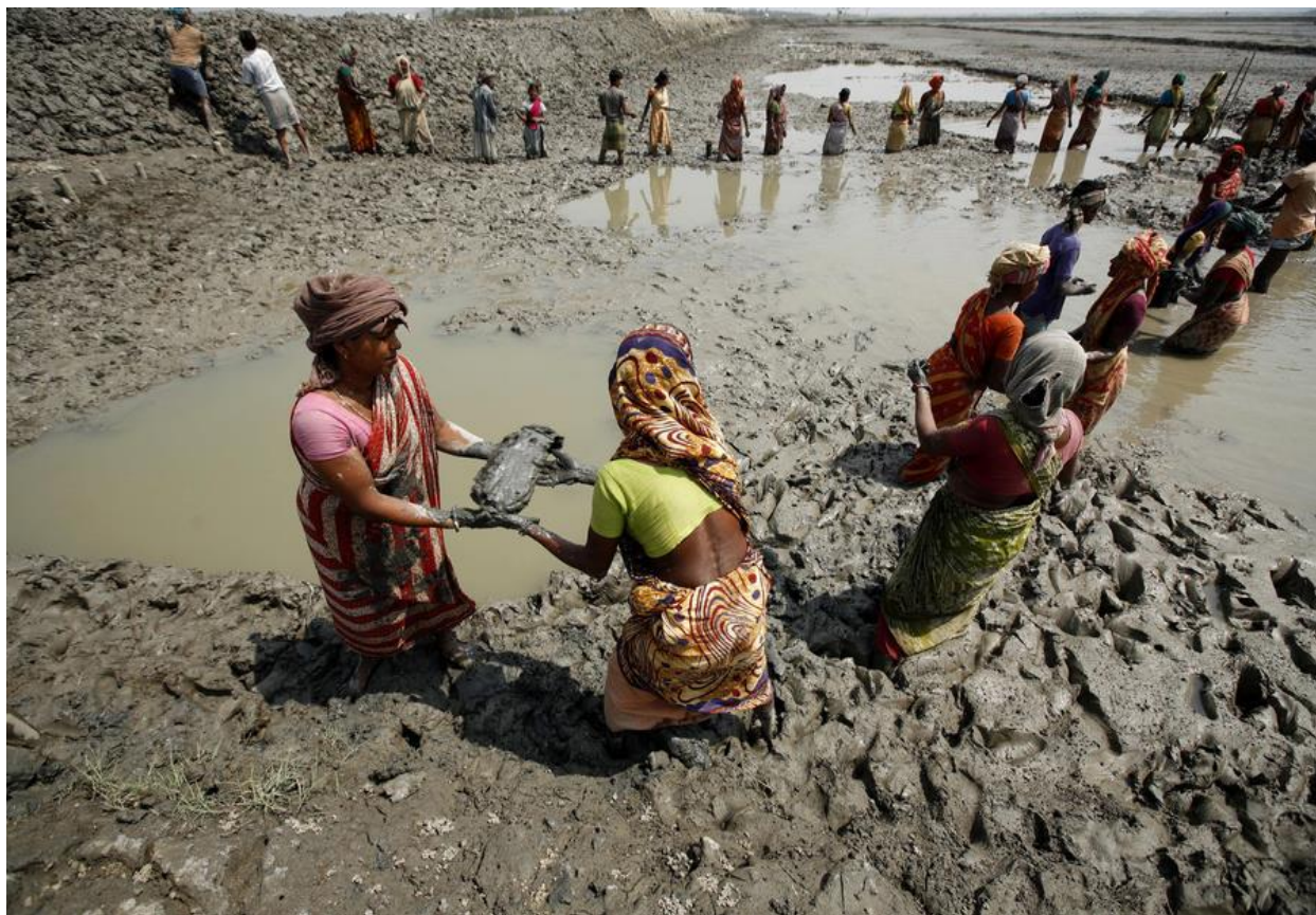
Figure 3: Women work to rebuild an embankment in one of the regions hit by Cyclone Aila in Khulna. Abir Abdullah / IOM. 2010.
